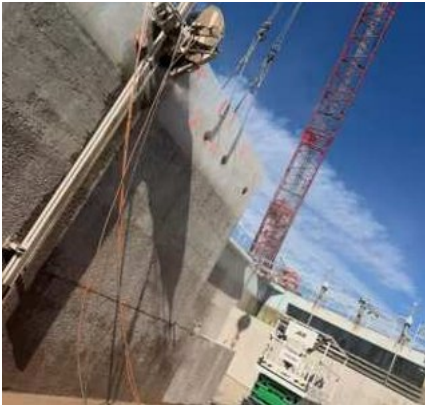
Rail-mounted wall sawing
