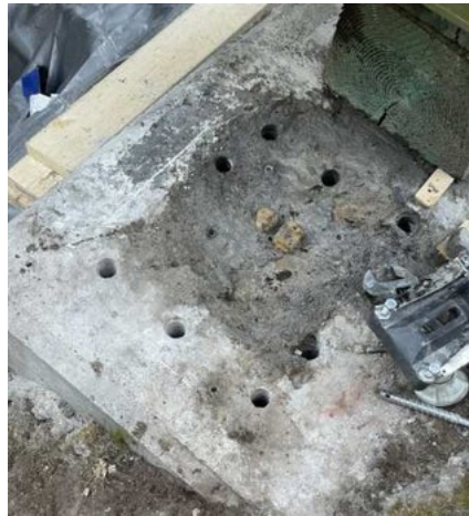
Drilled anchor holes
