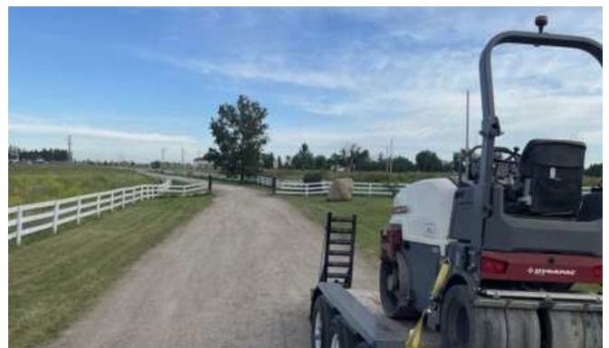
Driveway surface compaction
