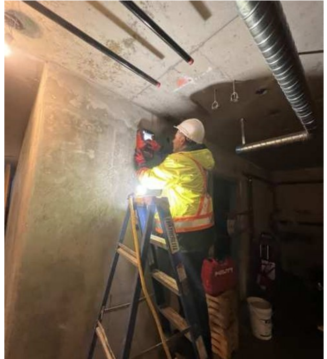
GPR scanning of concrete
