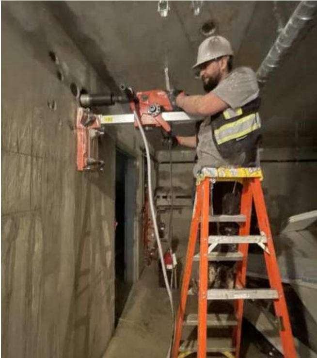
Wall coring in progress
