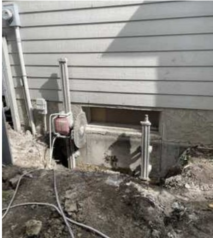
01 / Window opening cutting
