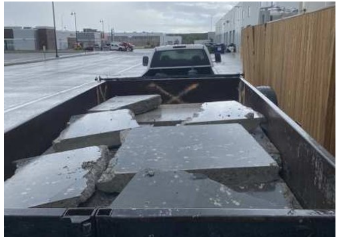
Removed concrete loaded for hauling
