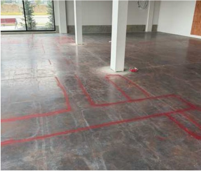
Before cutting: marked floor
