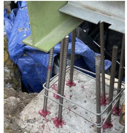
Rebar anchoring
