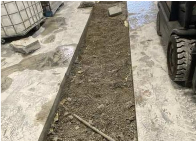
Concrete trench removal
