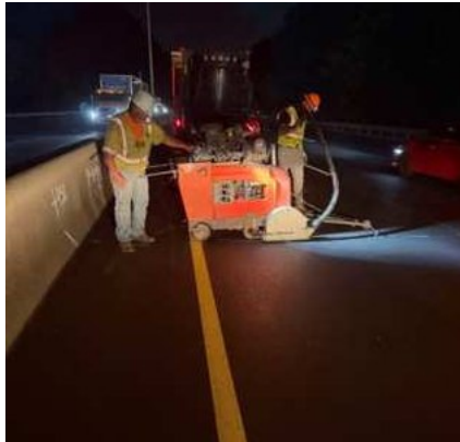
Asphalt floor sawing
