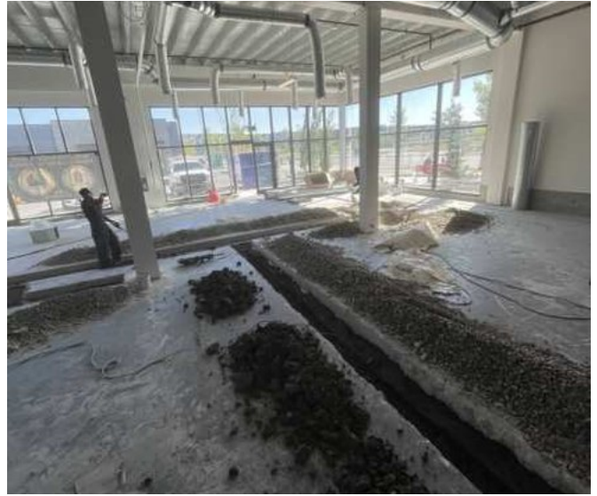
After cutting: opened trenches
