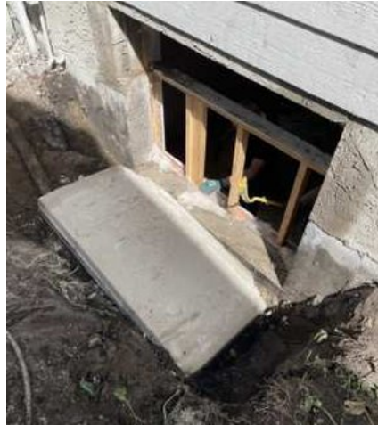
02 / Concrete section removed
