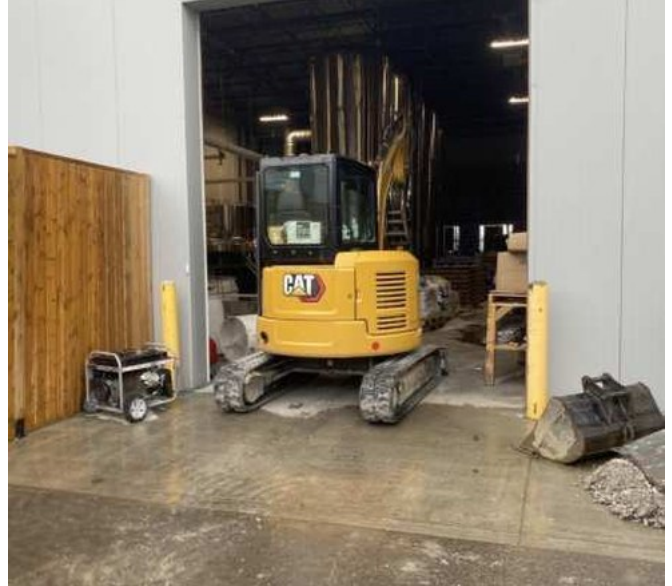
Excavator access for removal
