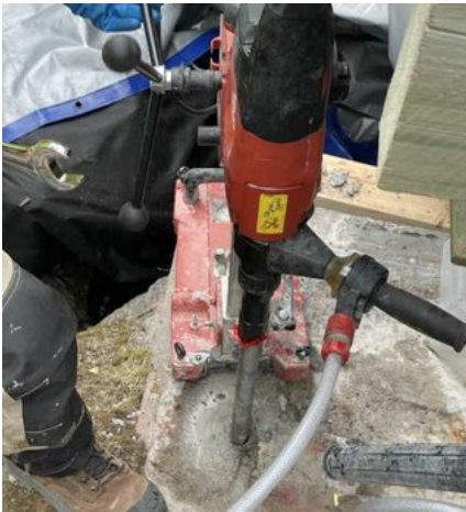
Concrete & Rock Coring
