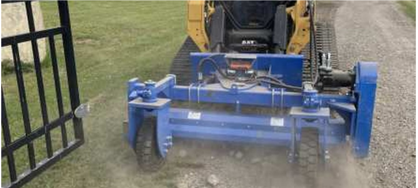
Power raking and driveway surface preparation
