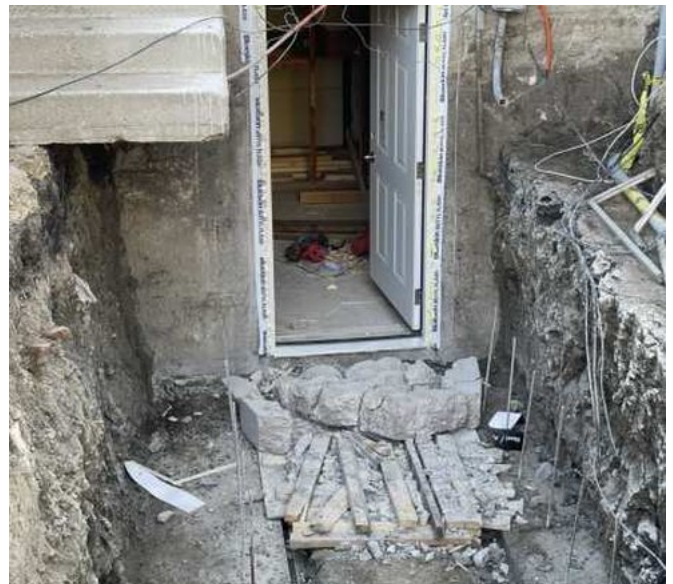
Door installed - work in progress
