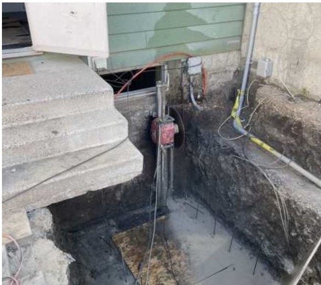
Cutting the foundation opening
