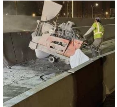
Concrete barrier cutting
